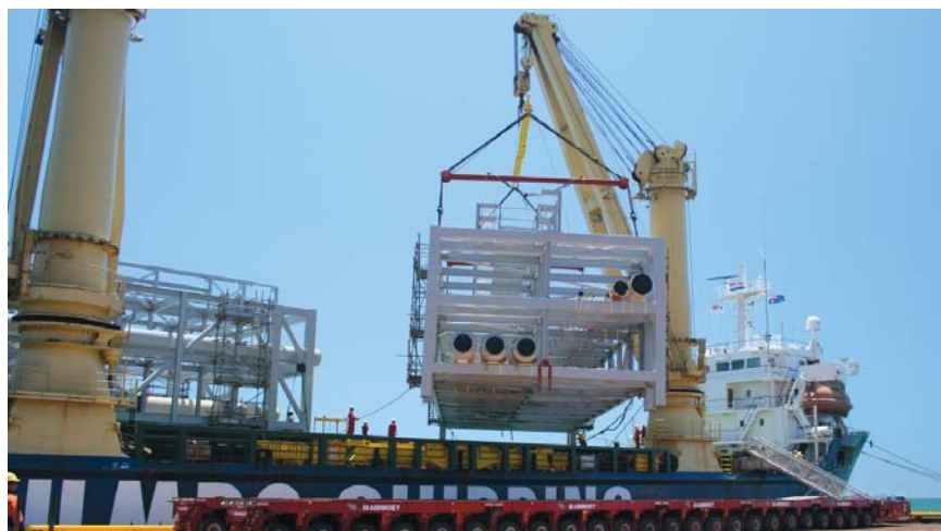
The first modules for Pluto's LNG train are unloaded
