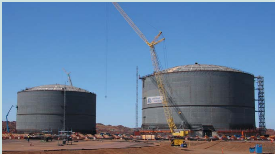
Pluto's LNG storage tanks take shape
